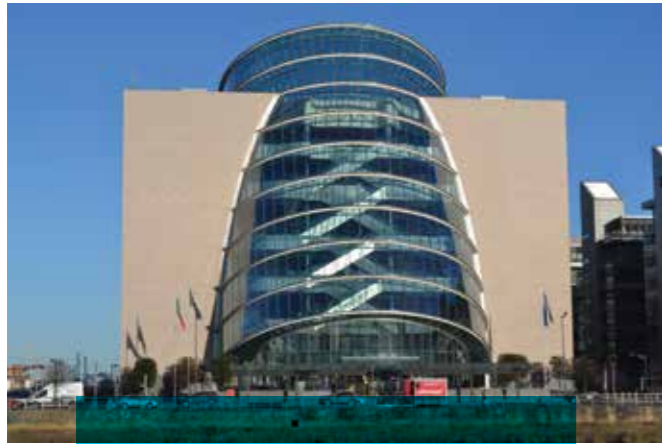
The convention centre Dublin – worlds first carbon neutral convention centre specified 70% GGBS
